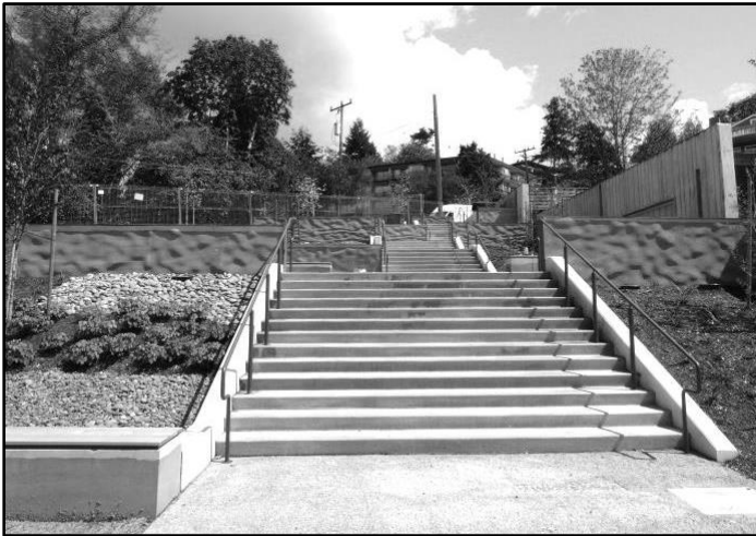
The public staircase links visitors to the viewpoint on the stormwater storage tank's green roof with Lowman Beach Park. Photo courtesy King County
