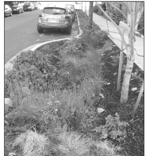
Rain gardens such as this along residential streets up the hill could retain water where it falls. Photo courtesy King County
